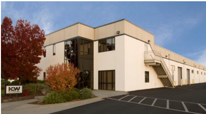
Kingsley Building: Administration, Information Technology, Engineering and Manufacturing
