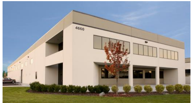
Grumman Building: Assembly and Shipping
